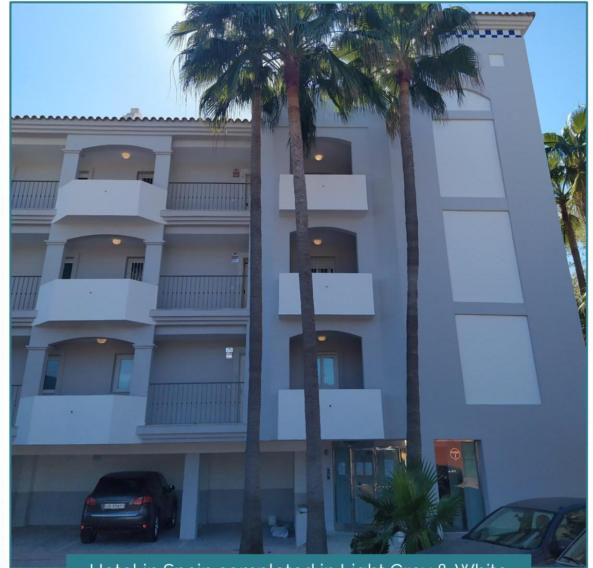
Hotel in Spain completed in Light Grey & White
